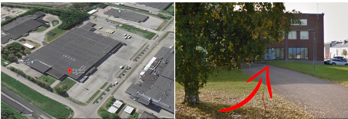
Figure 9.2. Location (N 65° 36' 43.558", E 22° 7' 56.554") and main access to the ICE Data Center.
